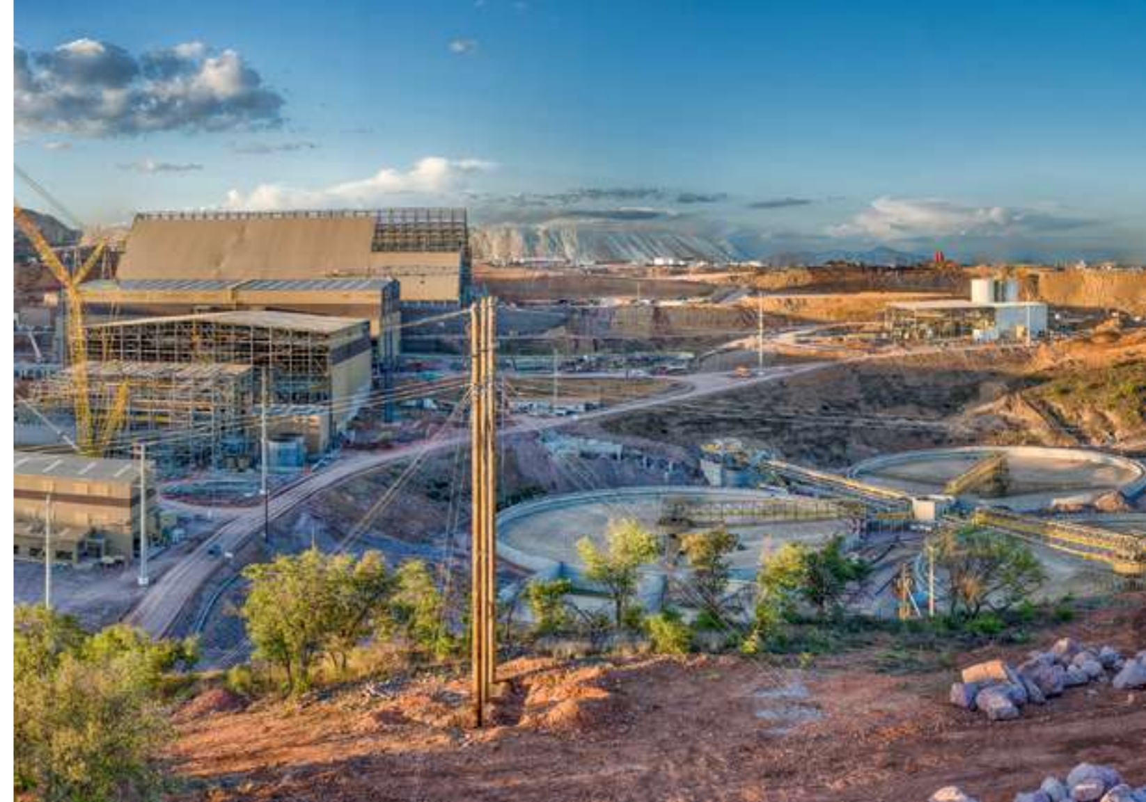
Concentrator II under construction at Buenavista del Cobre, Sonora, Mexico.
